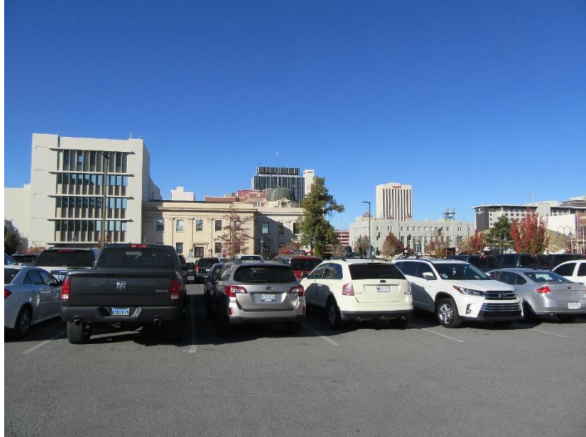
Photo Depicting Lack of Perimeter Fencing - Pioneer Parking Area
