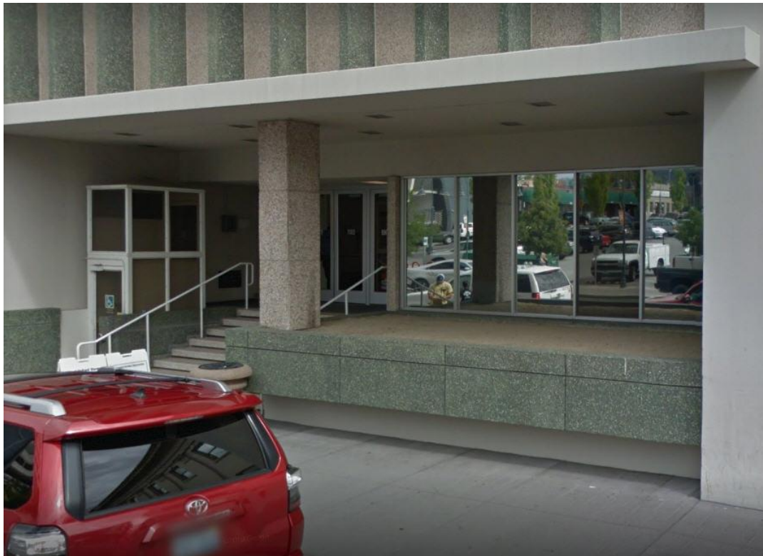
Location of ADA Accessible Lift – 75 Court Street
