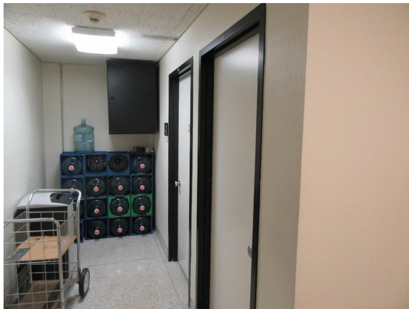
Figure 2-10 Photo of IT “Pull Box” Accessible to Public from Hallway
