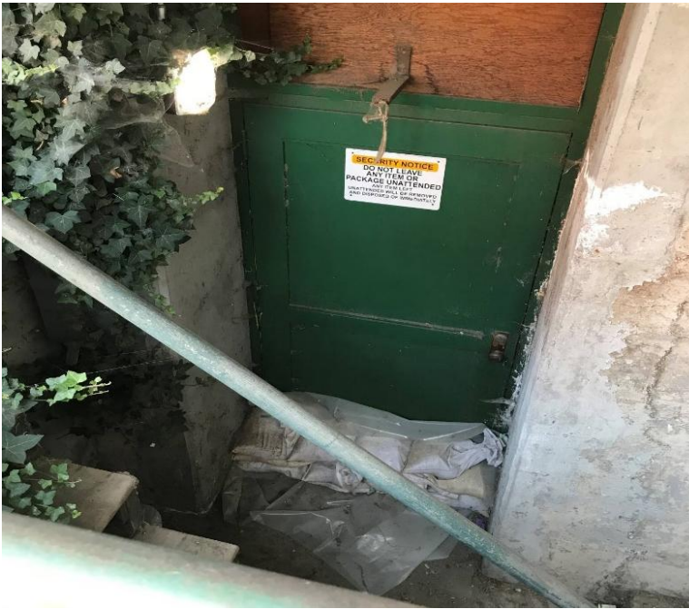
Figure 2-5 Basement Sandbags to Prevent Water Intrusion from Flooding – 75 Court Street
