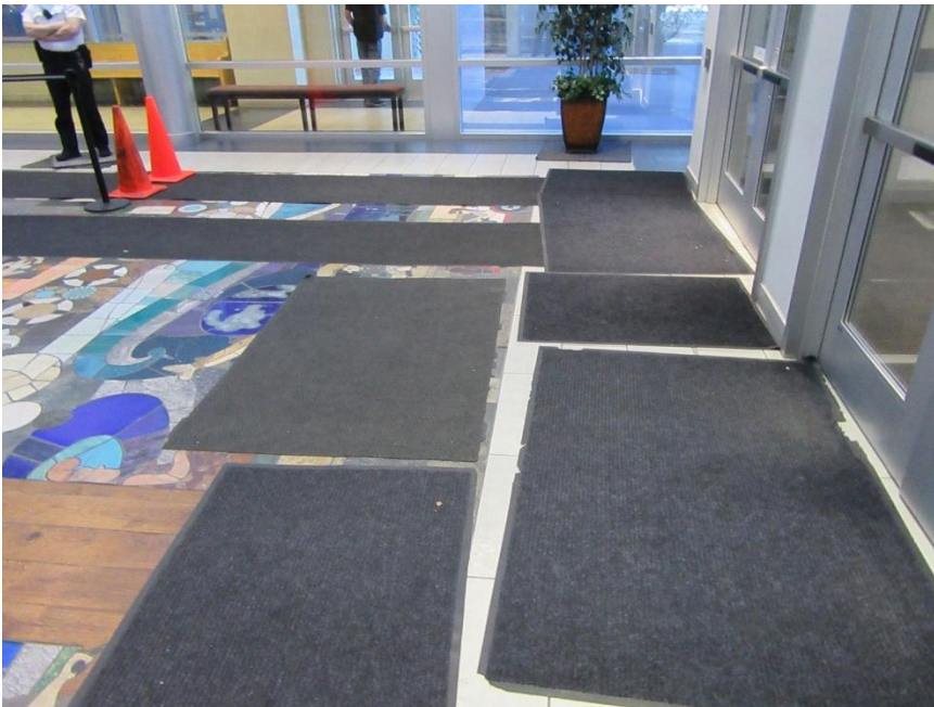
Figure 2-18 Photo of Main Entry/Screening Area – 1 South Sierra
